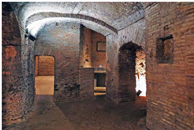
A possible wine cellar in the Case Romane. The original brickwork dates from the 3rd Century but later changes can be seen as the property eventually became one single dwelling
